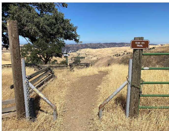
Photo 6. RMA boundary gate with trail width limiter for single track areas and Stay on Trail signage.
