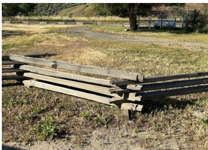
Photo 3. Split rail fencing used to restrict OHV access to closed riding area.
