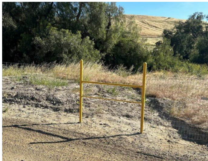
Photo 2. H brace used in fencing sections to allow wildlife passage.
