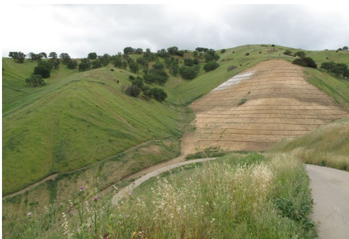
Photo 3. View of hillside erosion control in SRI Loop RMA from SRI Road.
