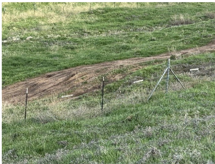
Photo 1. Field fencing with reflectors to enhance visibility of the fence.
