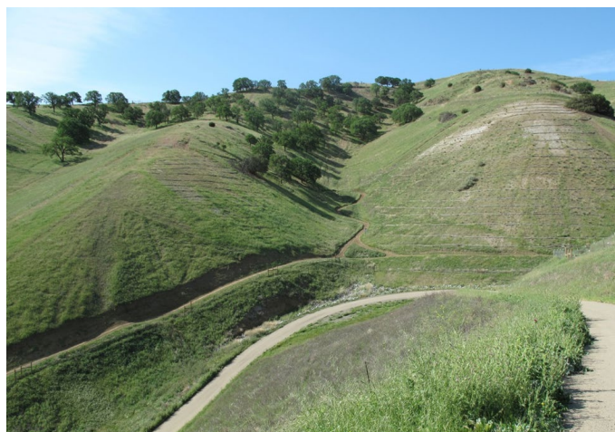
Photo 4. View of completed hillside rehabilitation in SRI Loop RMA from SRI Road.
